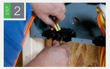
Slide the wire into the slot
